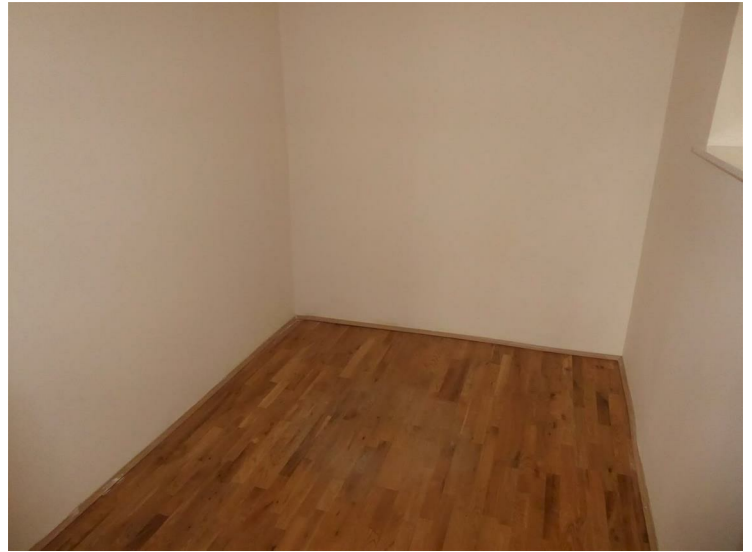
Front aspect double glazed window, radiator, power point.
